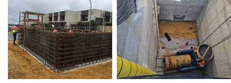
construct the access chambers. The open cut section of the works combined the use of proprietary shoring boxes, steel plates, benching and steel universal columns to support the excavations and services.
