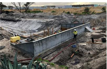
The project required a new pipe crossing to be installed under Scarborough Beach Road. The options to undertake the work were through open excavation or under-road boring to keep the road open. Several factors made it impossible to successfully bore the pipes, such as existing ground conditions, depth of cover to pipe and the closeness of each pipe to one another.
