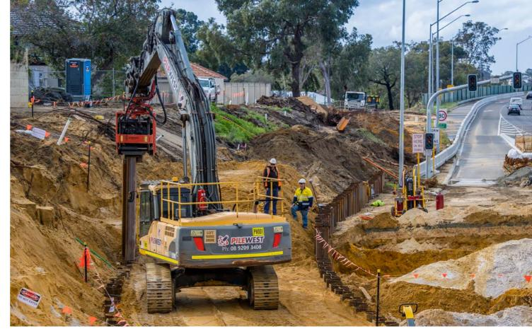
to provide further protection to the main, whilst the rest of the scope of works was undertaken. As an additional measure, ground vibration monitoring was used throughout piling works near the main to ensure no vibration limits were exceeded.
