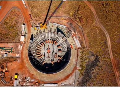
A concrete roof was installed on the water tank to ensure the design life is achieved and water quality is secure from any contaminates. The roof design used a hammer head style beam, which reduced the overall depth requirement and allowed for simplified construction with a single pin connection at the columns. Precast roof panels were then used to reduce formwork and provide a base for the final topping slab stitching the roof together.
