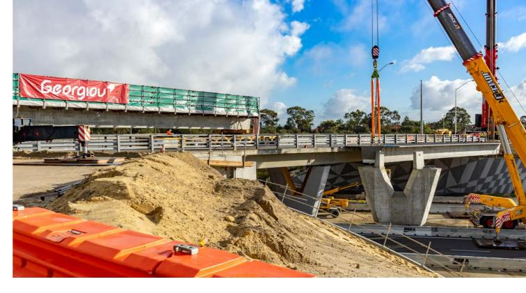
A significant consideration during the design phase was the interface with live services. To the south of the bridge, there was a high-pressure APA gas service and a BP fuel line servicing Perth Airport from Henderson. These two assets required significant interface with the relevant stakeholders for excavations, piling installation works and beam installation whilst traversing the assets.
